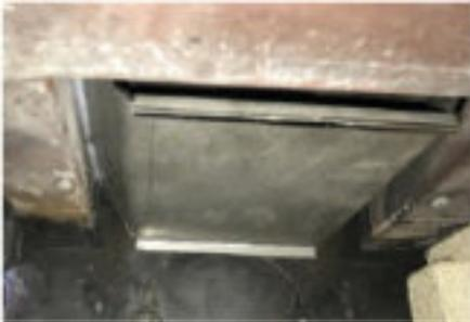
Remove upper steel baffle by lifting baffle off securing tabs. Slide to rear and push to right. The left side will now come down. Remove baffle.
