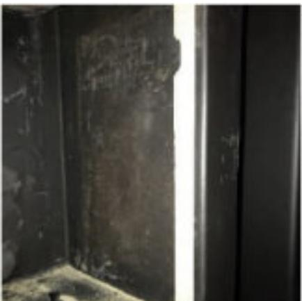
Remove side right and side left front bricks
