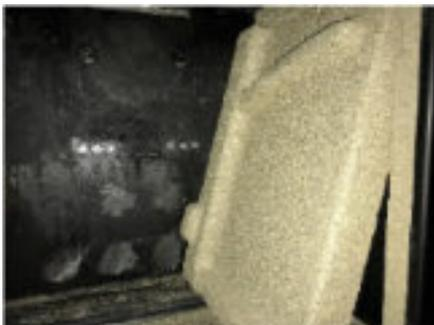
Remove side right brick baffle, take care as the upper side brick will come down when the brick is removed.
