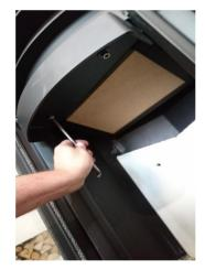
Using a 5mm hex key, unscrew the second baffle and it's bracket being careful to support its weight whilst removing.
