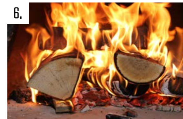
6. On the first light, the curing fire should be kept alight for 4 hours at a maximum temperature of 100°C to dry any excess moisture. On the second light, you need to increment the temperature of the oven gradually to temper the clay. From 0°C to 100°C and hold for 2 hours, from 100°C to 200°C and hold for 2 hours, from 200°C to 300°C and hold for 2 hours, from 300°C to 400°C and hold for 30 minutes and finally from 400°C to 500°C and hold for another 30 minutes. The last increment is the one that fully cures the oven and helps stretch your oven's performance capability.
