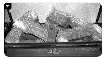
7.24 Once the logs are in place sparingly spread an amount of the Embaglow fibres provided on the sections highlighted, see Diagram 32.
