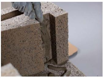
Press one side block into place and apply the lip glue into the slot as shown.
