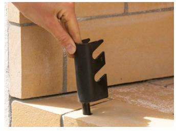
Drill  $2 \times 12$ mm diameter holes in the front row of the firebricks. Push log retainer holders in place.
