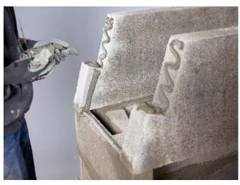
Apply lip glue to the joints on the sides of the front and rear panels of the gather.
