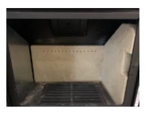
It is now possible to remove the top baffle brick by Lifting up the Left side and sliding it to the Left then dropping it down. The right hand side brick can be removed by gently pulling it down from the top.
