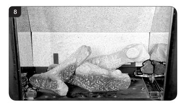
7.6 Place the foot of Log C into the rear left hand corner. The long flat edge rests against the side of the firebox and the log touches the back panel. The top of the log rests on Log E, see Diagram 9.
