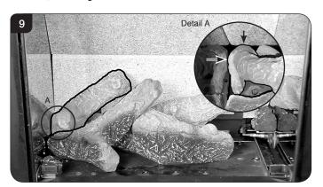
7.7 Place the pointed bottom of log D into the corner of the burner tray and rest on the location stud on log B, see Diagram 10.
