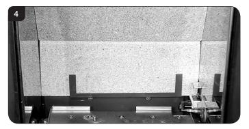
7.2 Place Log A on the higher rear bracket and push up against the back panel, see Diagram 5.
